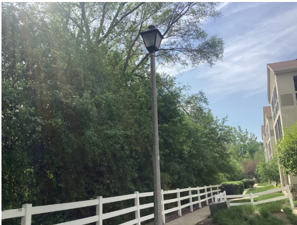
Light pole and fixture
