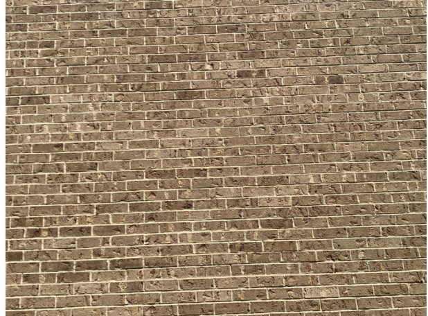
Masonry walls overview
