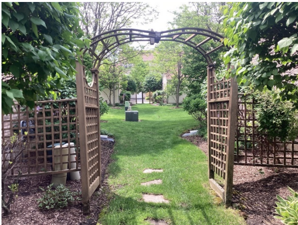
Trellis overview – note sag in center
