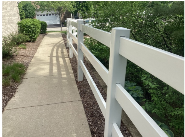
Vinyl fence overview – note slight lean
