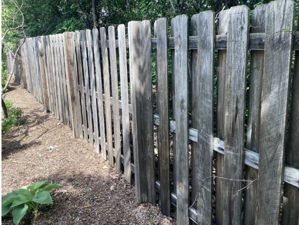
Wood fence overview
