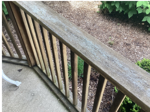
Railing – note organic growth
