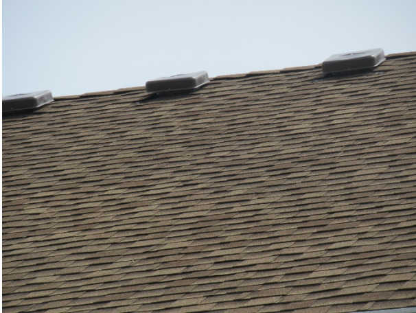
Roof overview – note square hood box vents
