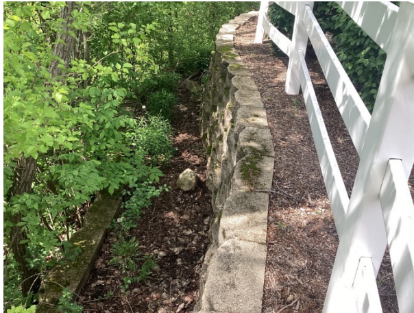
Masonry retaining wall – note organic growth
