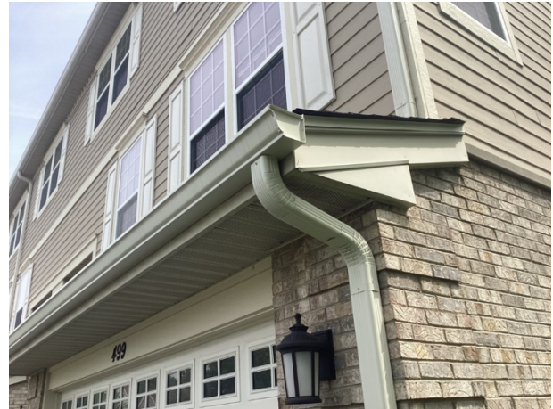
Typical gutter and downspout configuration
