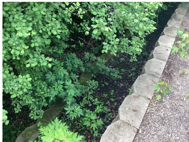
Tiered retaining wall
