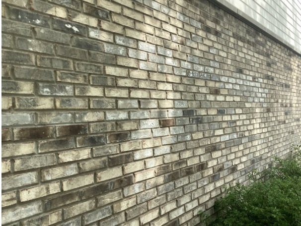
Masonry walls overview – note slight efflorescence
