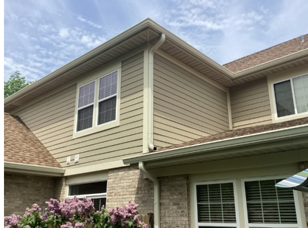
Typical gutter and downspout configuration – note downspout discharges directly to roof
