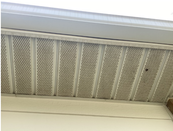
Soffit and fascia overview
