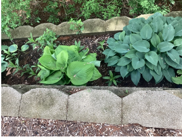
Tiered retaining wall
