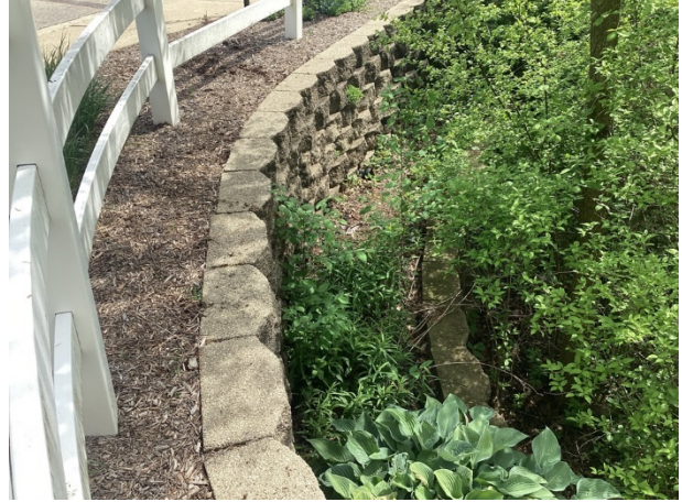
Masonry retaining wall overview
