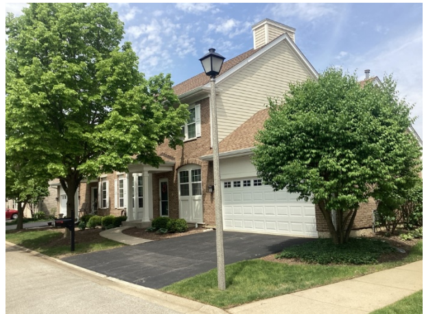
Light pole and fixture
