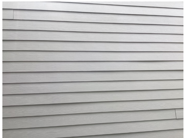
Fiber cement siding overview
