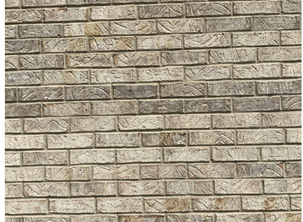
Masonry walls overview
