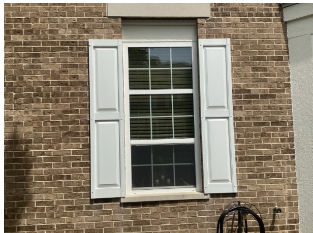
Vinyl shutters overview
