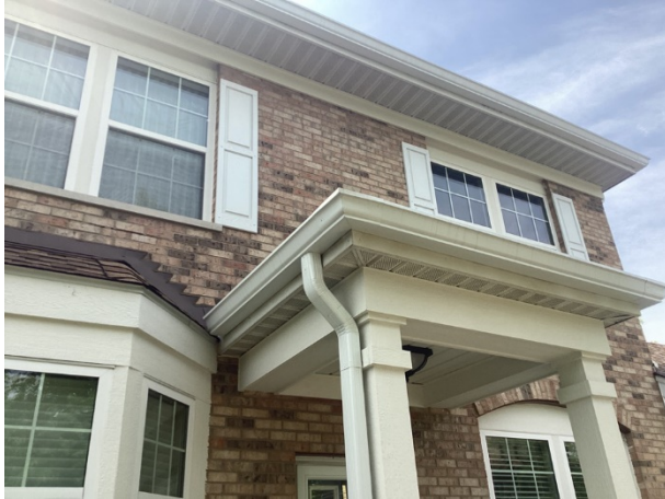
Typical gutter and downspout configuration
