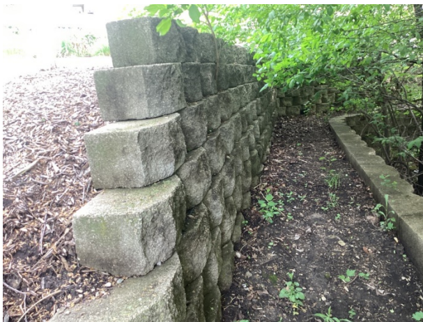
Retaining wall overview
