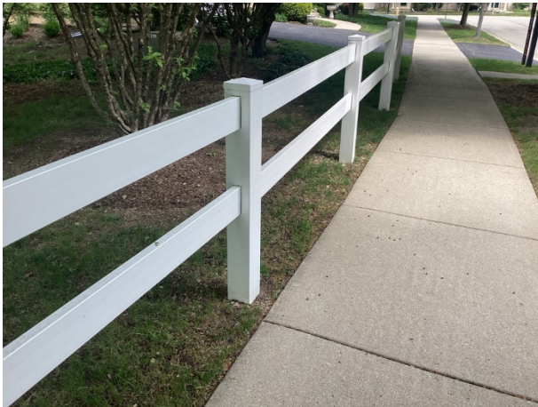
Vinyl fence overview
